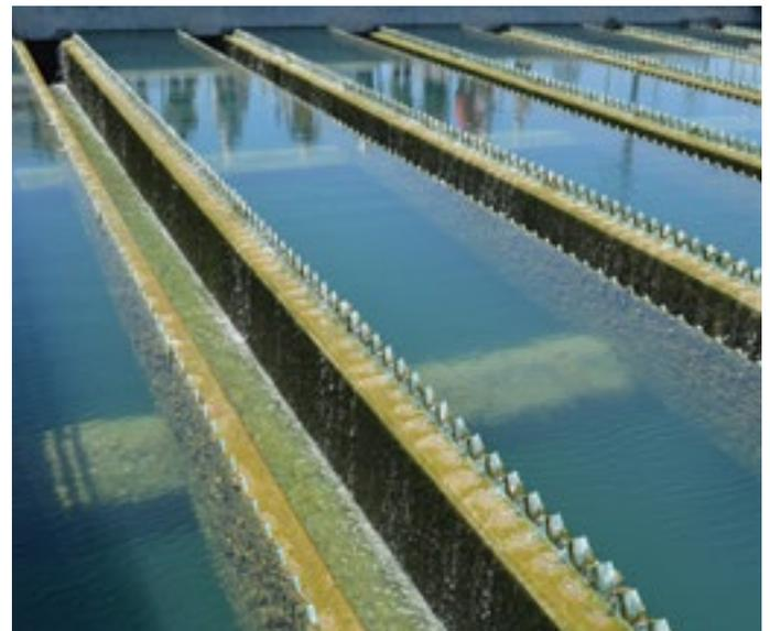
Sedimentation basins at Randall-Bold Water Treatment Plant remove many particles from the water.
