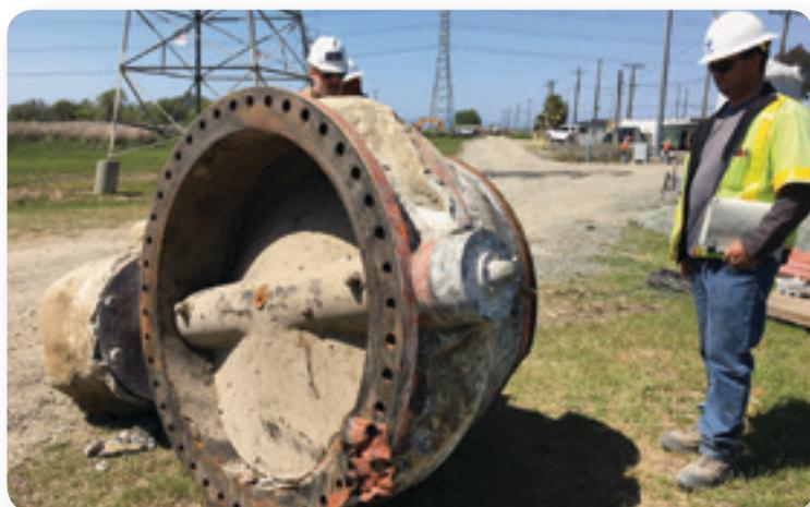
Crews inspect an old 48-inch valve that was replaced while upgrading the Shortcut Pipeline.
